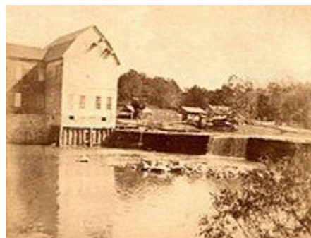
Sly Mill, a grist and saw mill on Spring River in the Springfield Plateau, c. 1860
